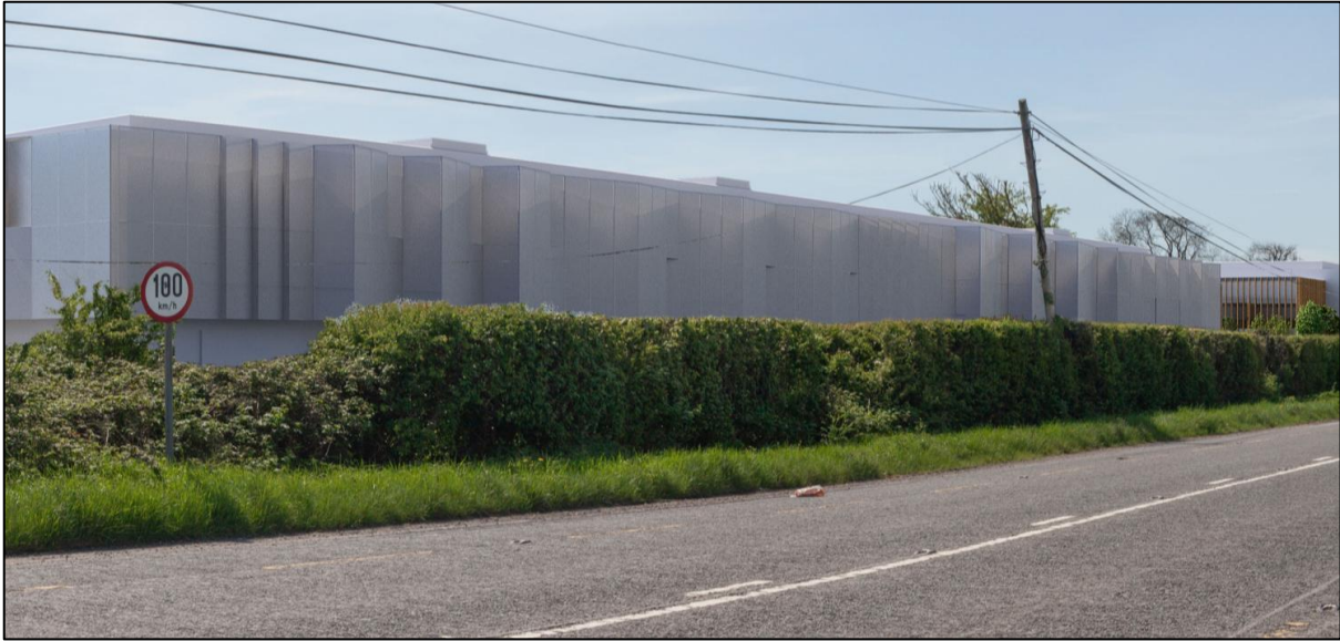
Figure 4: Proposed metal veil on the R446 facing side of the proposed data halls
